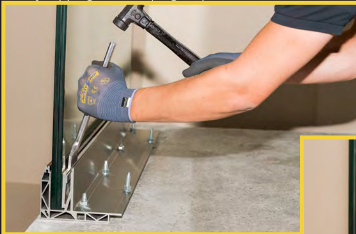
Gently tapping the clamping strip
