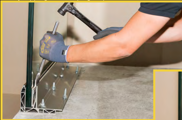
Gently tapping the clamping strip
